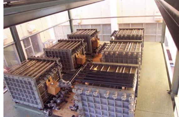
Fig 6. Upper level of VRB
